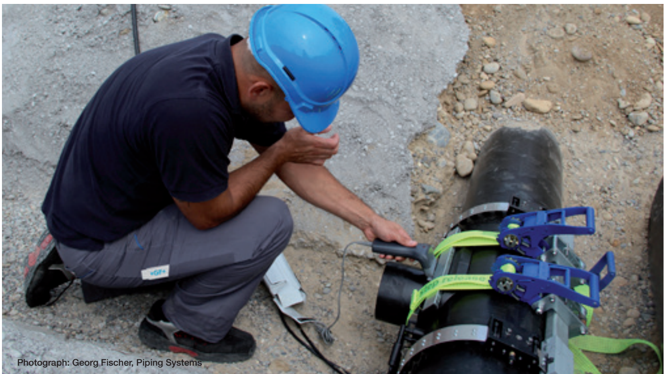
Fig. 2: Practical example of a saddle weld by means of electrofusion welding.
