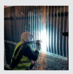
Twin Arc Spraying (TWAS) Laser Cladding
